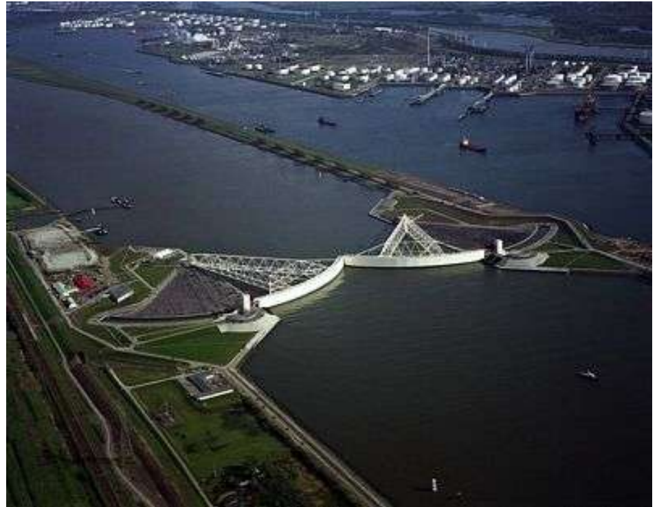
Deltaworks in the Netherlands
